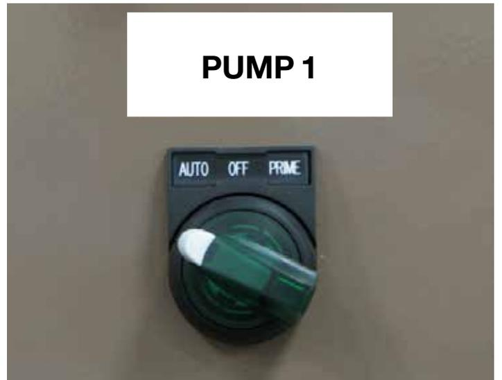
**Step 10:** Then turn PUMP #1 Switch to OFF position. Repeat this rinse process for each Pump used (1-4).
