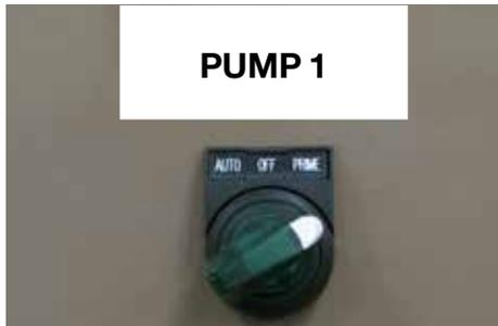
**Step 9:** Turn Pump #1 Switch to OFF position.
