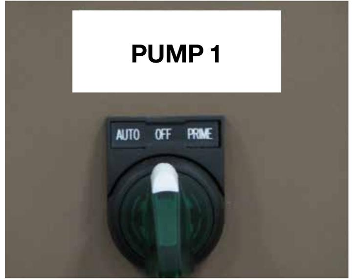
**Step 7:** Turn the RH Basic PUMP #1 Switch to the AUTO position. Allow the Pump to run and completely empty the CBP Tank, Pump Element, Treatment Line.
