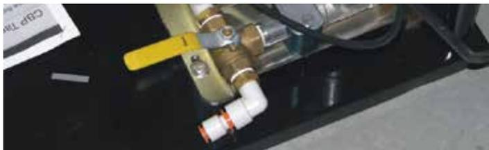
**Step 4:** Ensure the tank valves are in the TREAT mode.
