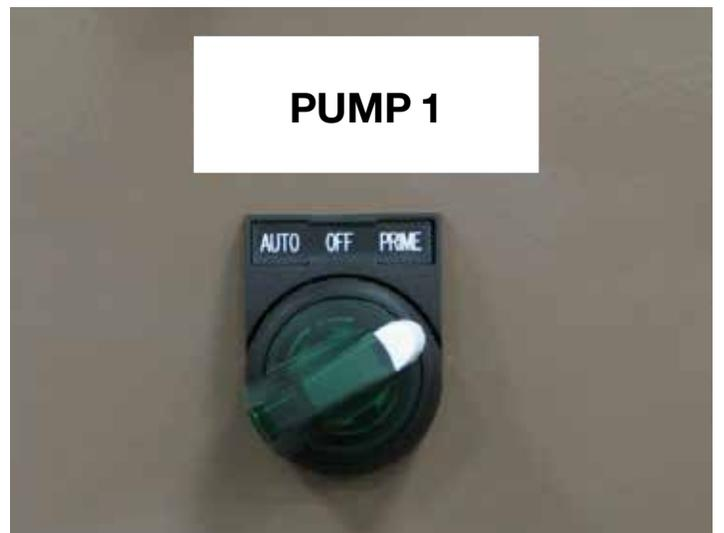
**Step 7:** The Pump will run, purging the treatment lines of air and send chemical to the Treater Chemical Inlet Assembly.
