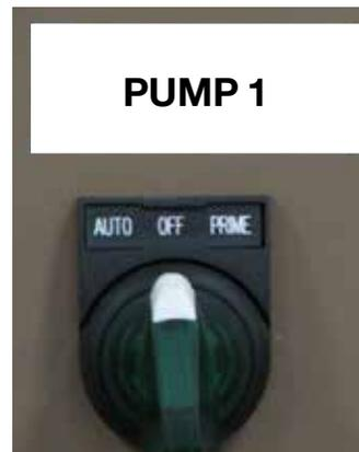
**Step 8:** Turn the RH Basic PUMP #1 Switch to the PRIME position.
