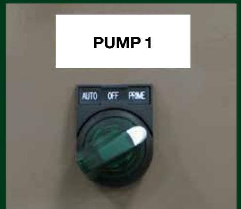
**Step 6:** Turn Pump #1 Switch to OFF position.
