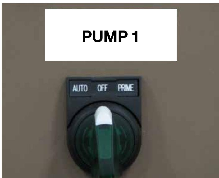
**Step 15:** Turn the RH Basic PUMP #1 Switch to the PRIME position.
