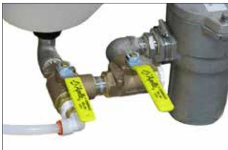
**Step 2:** Check filters periodically for clogging issues. Use a 9/16" wrench to remove the filter cap from the filter body. Remove the filter basket and clean thoroughly.
