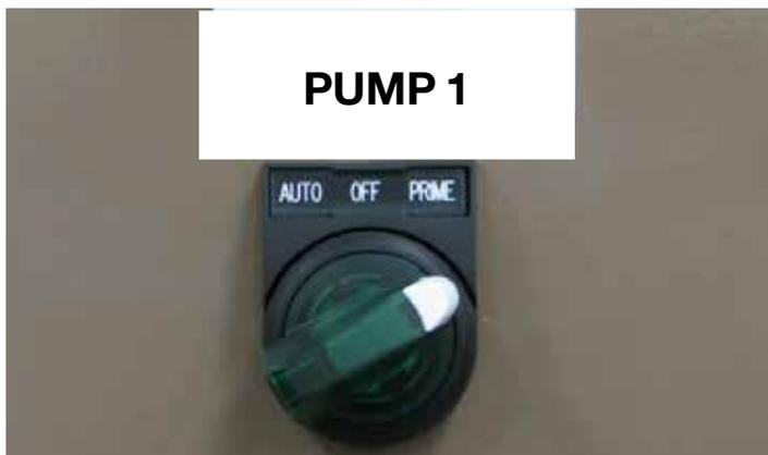
**Step 22:** The Pump will run, purging the treatment lines of air and send chemical to the Treater Chemical Inlet Assembly.
