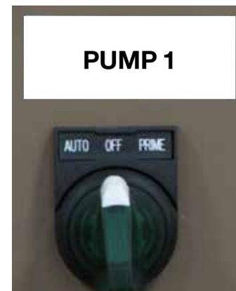
**Step 11:** Turn the RH Basic PUMP #1 Switch to the PRIME position.
