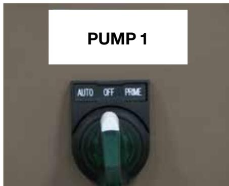
**Step 14:** Turn the RH Basic PUMP #1 Switch to the PRIME position.
