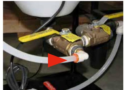
**Step 13:** Cut to fit and connect the other end of the Transfer Tube to the Press-lock Fitting underneath the Flow Meter.
