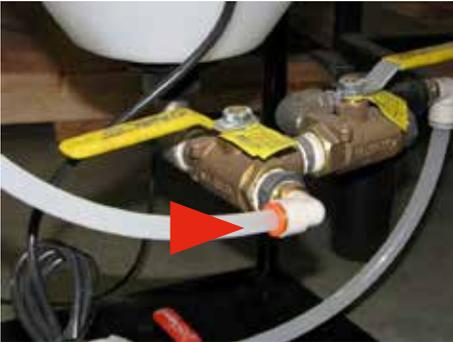
**Step 13:** Connect one end of the Transfer Tube to the Press-lock Fitting on the pump, located underneath the CBP Tank.
