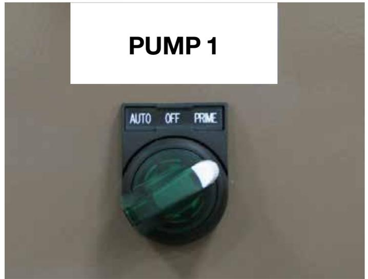
**Step 15:** The Pump will run, filling the Calibration Graduated Beaker with chemical for one minute.
