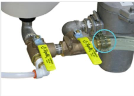
**Step 9:** Replace the 3/4" Pipe Plug on the Drain Valve. Use a crescent wrench to tighten in place.
