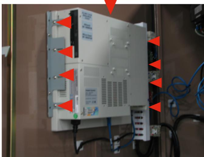
**Step 3:** Remove three brackets from the control panel door.
