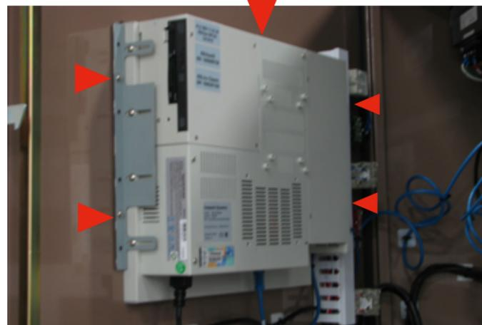
**Step 4:** Tip the existing HMI out of the front of the control panel and carefully remove it, holding on to it with your hand.
